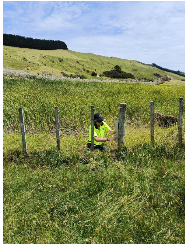
Installing ZIP Motolures December 2022
